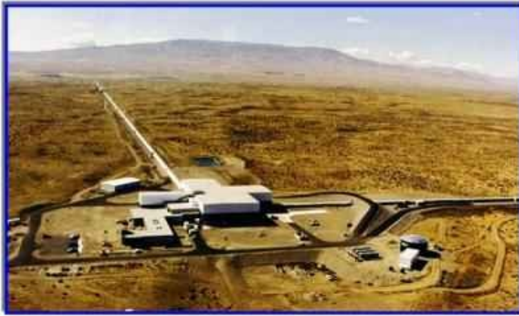
The 4 kilometer long, L-shaped, LIGO gravitational wave detector in Hanford, Washington [Photo used by permission of the LIGO Project, California Institute of Technology]
